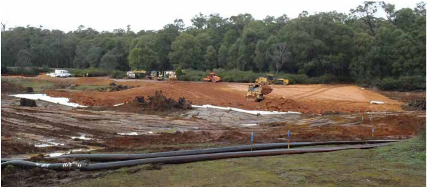
On 9 June 2014, Main Roads' contractors commenced preliminary construction activities at the Hamilton River site. Works included preparing access tracks, hardstand areas, stockpiling materials, as well as installing two coffer dams to aid with dewatering the site. Work was advancing well and the construction of the new culvert and embankment causeway had commenced when significant rainfall in the Hamilton River catchment resulted in works being postponed for winter.
